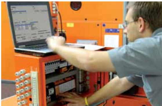
Plant diagnosis with state-of-the-art technology
